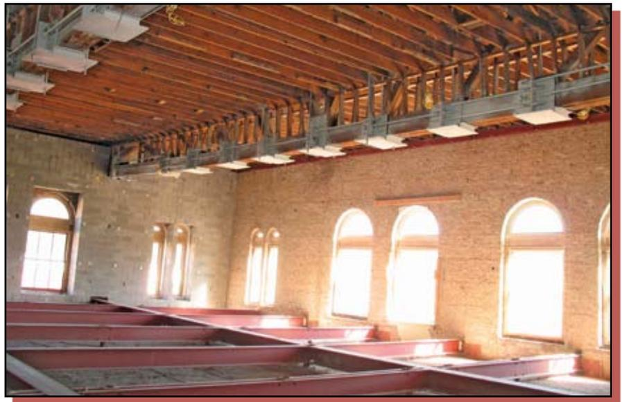
Figure 5: Repair of trusses and new floor framing in ballroom.
