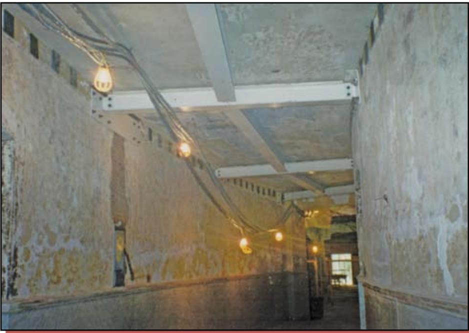
Figure 4: Typical floor framing repair in corridor.
